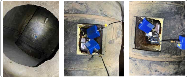
Installation of two specialized AE sensors and signal amplifiers on prepared DH pipelines for data acquisition
