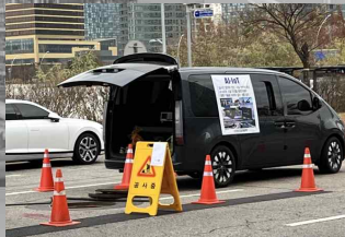
Field measurement scene showing the diagnostic equipment loaded onto a vehicle operating in an urban area, conducting tests at various manholes for district heating pipelines
